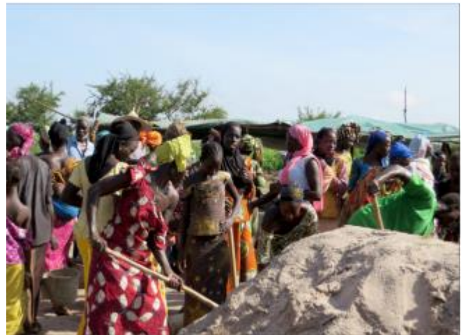
Photo: Women work at mixing cement on the work-site.
