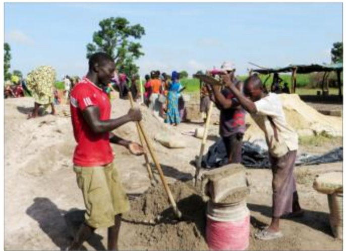
Photo: The community members make bricks for the school.
